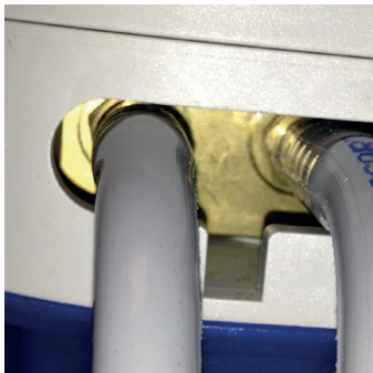
Figure 4: Access to ground
