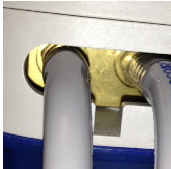
Figure 4: Access to ground
